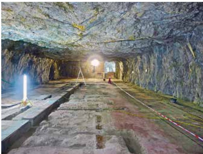
Admiralty Wireless Station. The floor pattern indicates extensive equipment, long since removed
